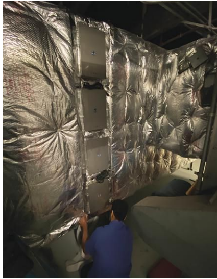
PLUG 'N' PLAY Air-treatment systems such as RGF Environmental Technologies' units are designed to be installed directly in the supply side of HVAC systems, with minimal disruption to building operations.
